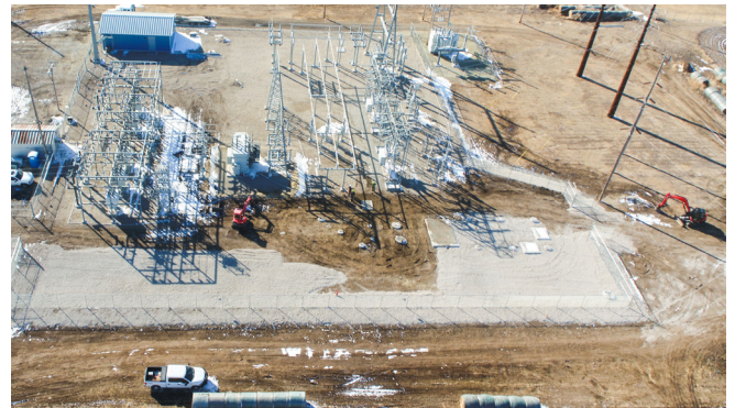
Images of the progress of the substation upgrade north of Phillipsburg at the end of February were taken by drone.
