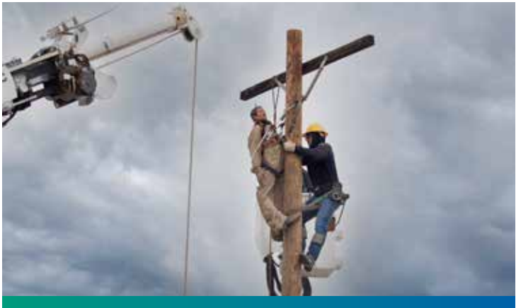
Pole top rescue training is repeated every year to drill this life-saving skill into all our lineworkers.
